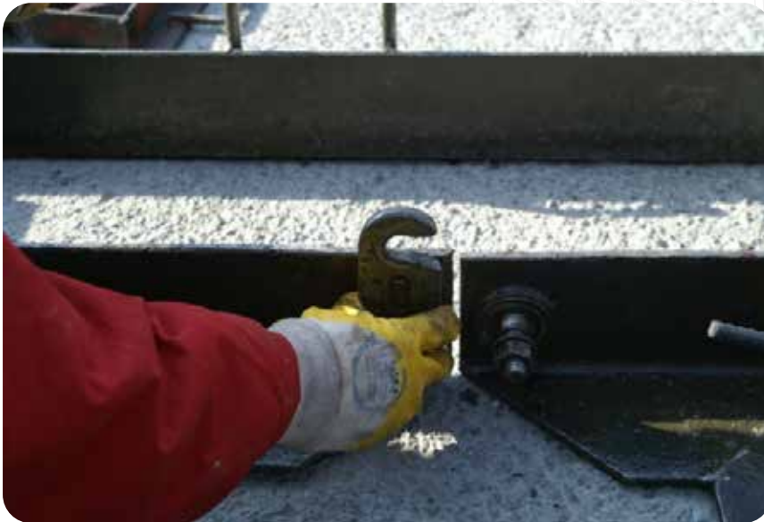
Fixing of threshold on concrete foundation surface
