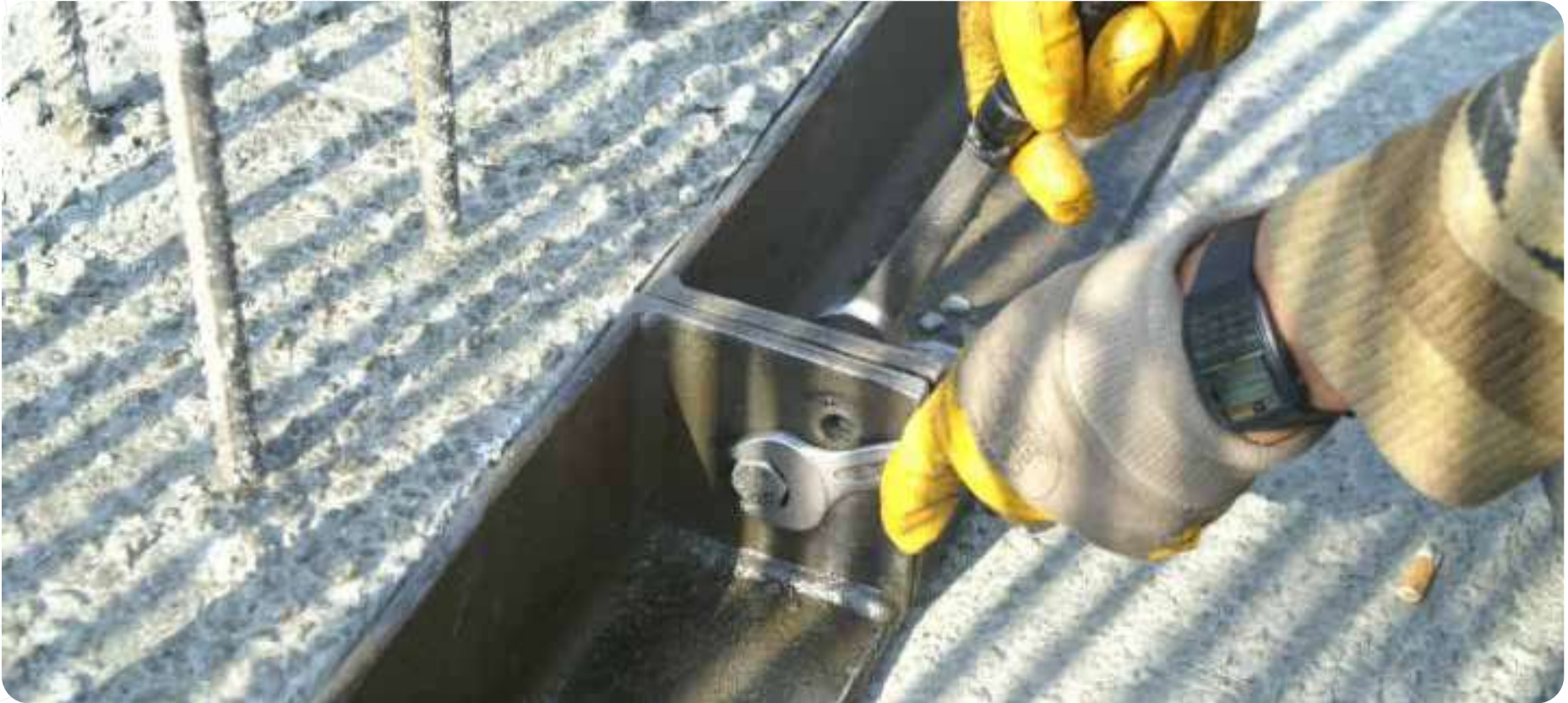
Threshold bolts removal
