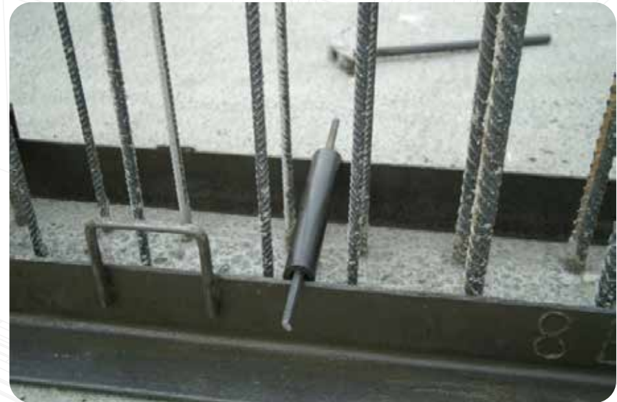
The cone spacer is used for wall thickness adjustment.
